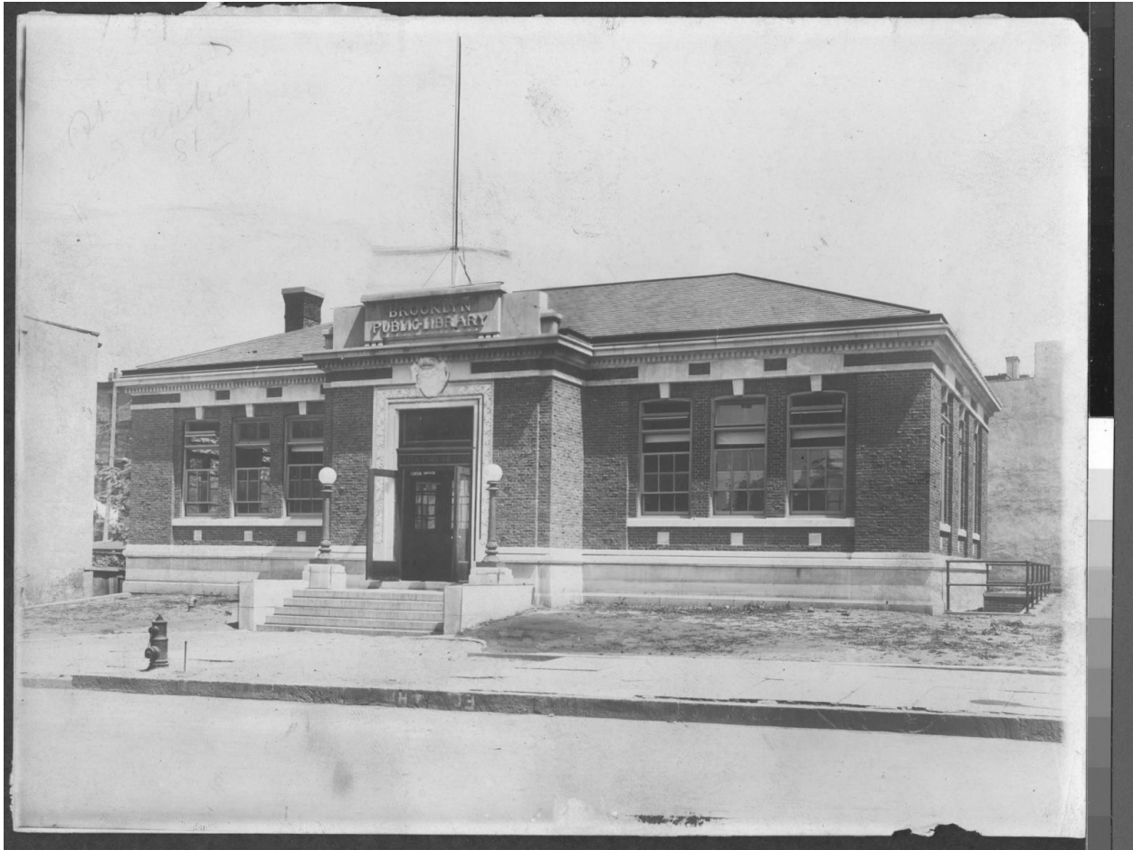
Archival photo Walt Whitman Library architect Rudolph I. Dass 1908
